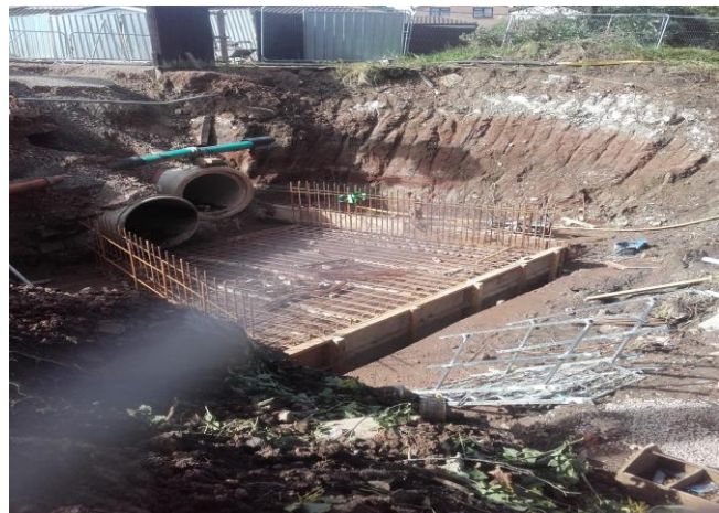
Image: Brookfield Avenue Culvert Crossing Works
