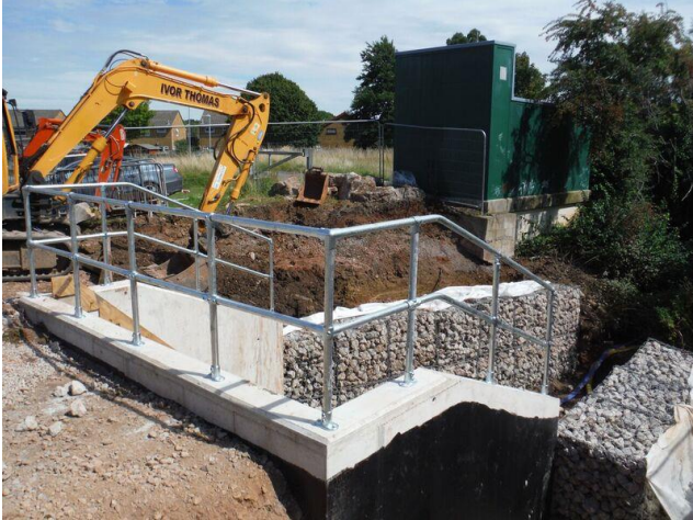
Image: Meadowvale Headwalls.
