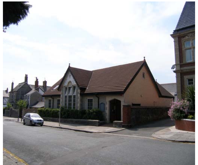
Alterations and improvements to extend community facilities at St. Augustines Parish Hall
