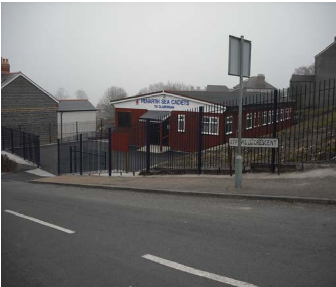
Refurbishment and Landscaping works to Penarth Sea Cadet Hall
