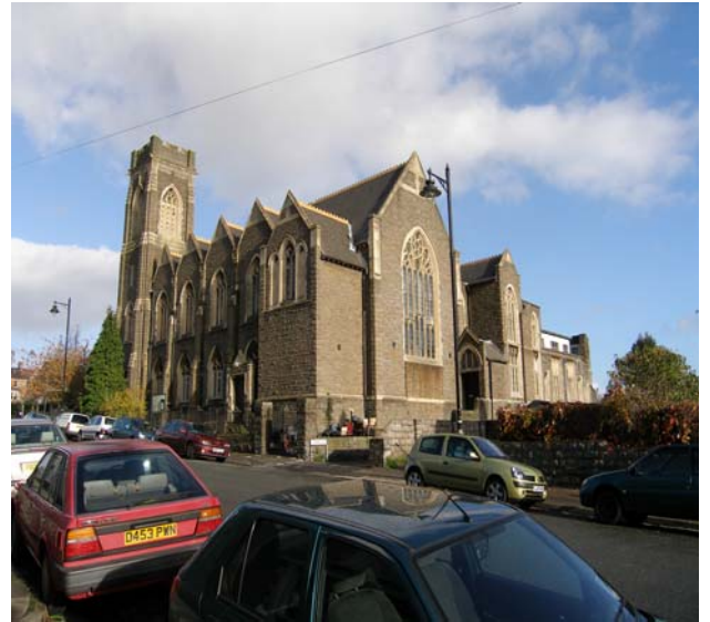
Refurbishment of basement to provide large, multi-use area especially for young peoples activities
