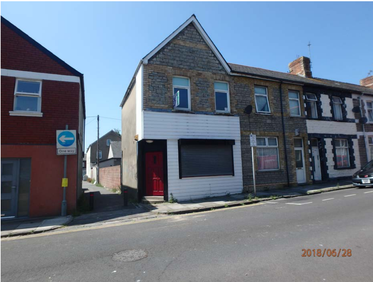
Site visit photograph
