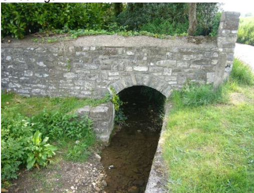
Bridge at Aberthin House
