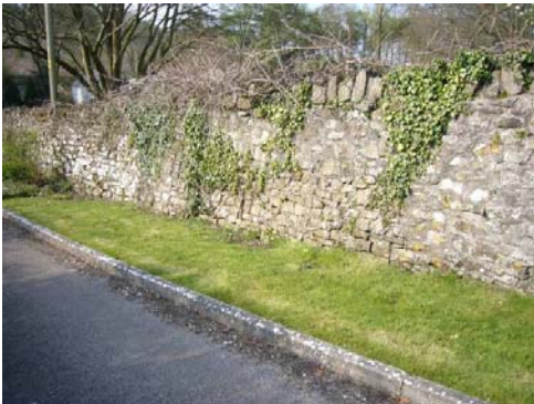
Stone walls are part of the area's special interest.
