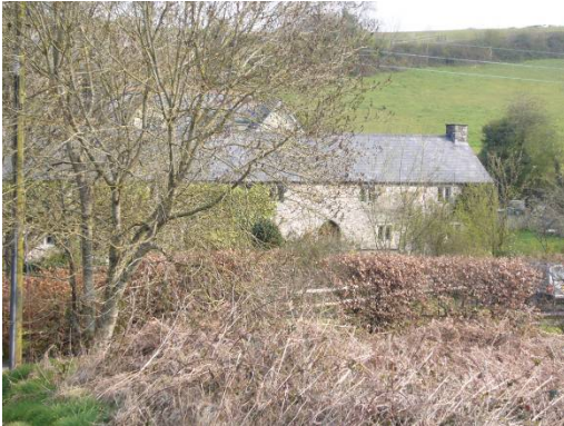
Range of Buildings at Court Farm
