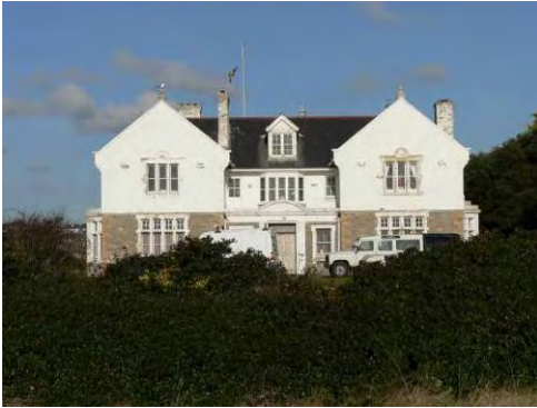
Friars Point House.
