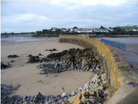
Old Harbour Breakwater.
