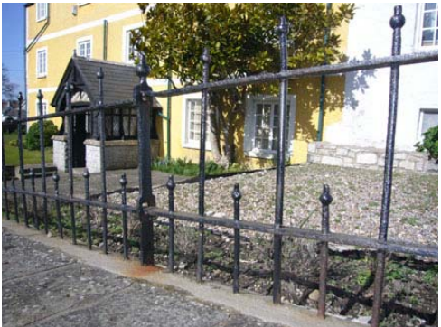
Garden Walls and Railings of Boverton House
