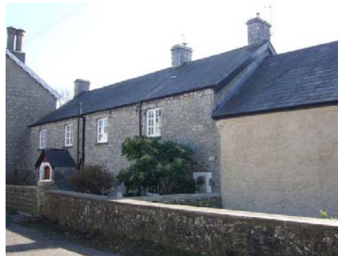
Orchard House Farm and attached farm buildings are now converted to residential use using appropriate materials.
