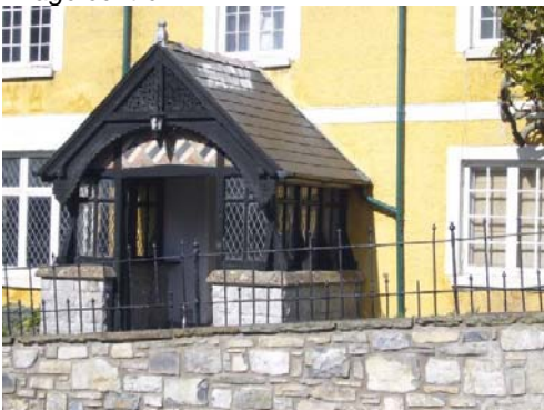
Porch and historic railings at Boverton House.
