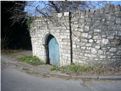
Walls Surrounding Garden West of Boverton House
