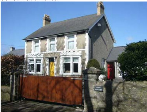
Cwrt Newydd, Boverton Road, though not listed this buildings makes a positive contribution to the conservation area.
