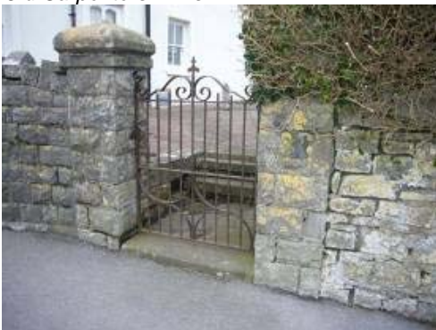
Stone gate piers and a decorative iron gate add to the local distinctiveness of the area.
