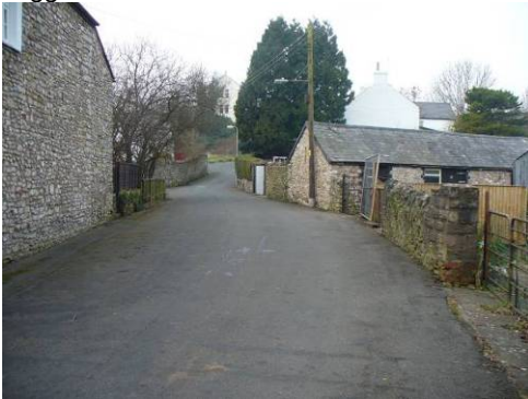
The rear wall of Yew Tree House provides enclosure to the lane.
