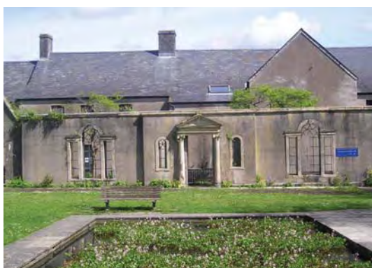
The remains of a once fine 18th Century facade is retained as a screen wall on the northern frontage of Old Hall Gardens
