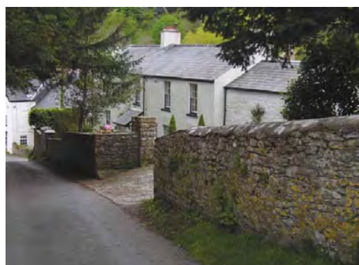
The Firs: a well preserved house of late 18th/early 19th century appearance, slate roof, sash windows and rendered rubblestone walls.
