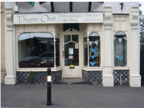
A well preserved and finely detailed early 20 th century shopfront at no. 5 Elm Grove Road.
