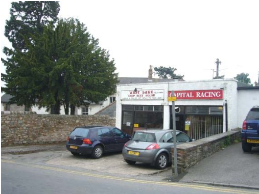
Flat-roofed single storey shops are out of keeping with the historic character of the conservation area.
