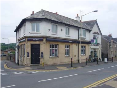
This large bank dating from 1914 indicates the importance of the area at the start of the 20 th century.
