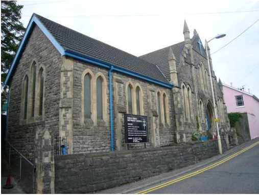
Methodist Chapel, Station Road
