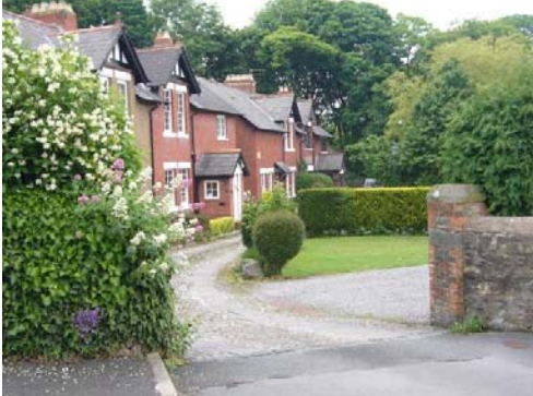
Late 19 th century houses contribute to the historic character of the village.
