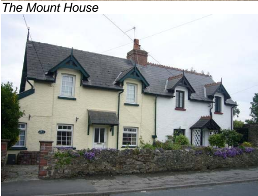
Holly Cottage (Right) and Mount Cottage (Left) are County Treasures.
