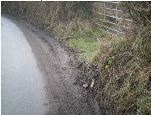
Some verges are being eroded.
