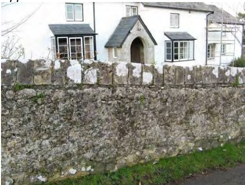
Stone walls outside Y Hen Fferm Dy.
