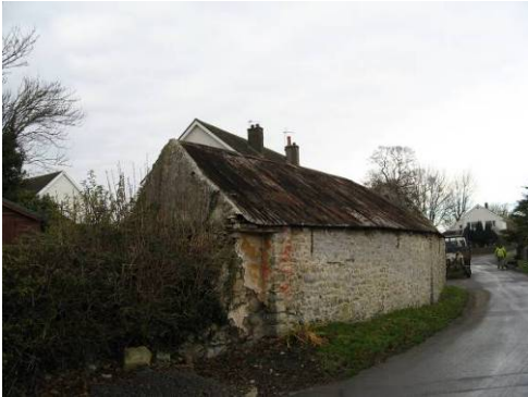
The derelict outbuilding on the east side of Ivy Cottage
