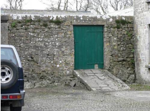
Kitchen Garden Wall.
