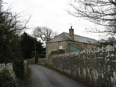
The listed stables and walls define the entrance to the Conservation Area.
