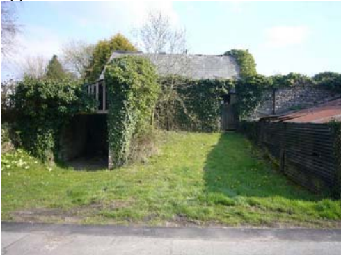
Ivy can be a cause of decay in old buildings.
