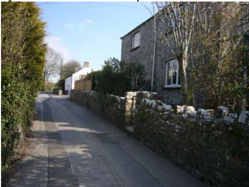
Railway Cottages were built about the same time as the arrival of the railway, 1897.
