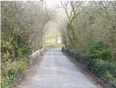
An 18 th century stone road bridge crosses Nant Llanmihangel.
