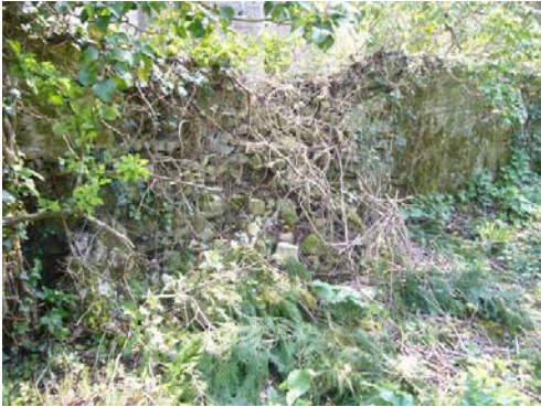
The churchyard wall is in danger of collapse in certain places
