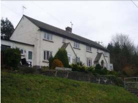
Goscombe Place, former rural district council houses.
