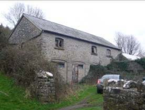
Two storey farm building.
