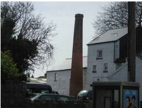
Chimney to former Oast House.
