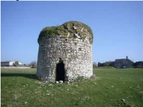
Medieval buildings at the site of the grange are in danger of falling into disrepair.
