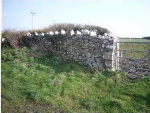
Stone walls and wide grass verges are a feature of the area. Walls are often topped with a 'cock and hen' coping.
