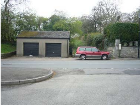
Modern double garage that is out of keeping with the conservation area.
