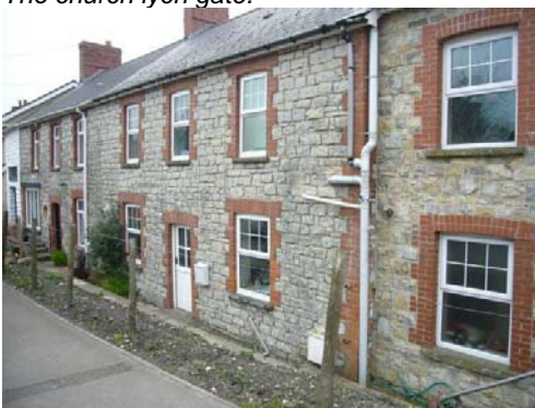
Local lias stone with red brick window and door dressings are typical of the area's 19 th century buildings.
