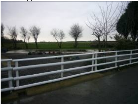
This timber post and rail fence is out of keeping with the stone walls or hedges that typically form boundaries.
