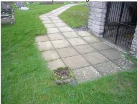
Concrete slabs are a poor quality surface for the approach to a medieval church.
