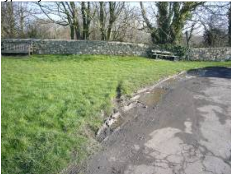
Car parking by the green is eroding the unkerbed grass verge.
