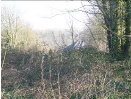
Trees and greenery usually obstruct views of the track across the viaduct.
