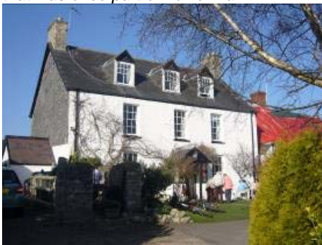
Lower Farm House is a grade II listed building dating from the mid/late 18 th century.
