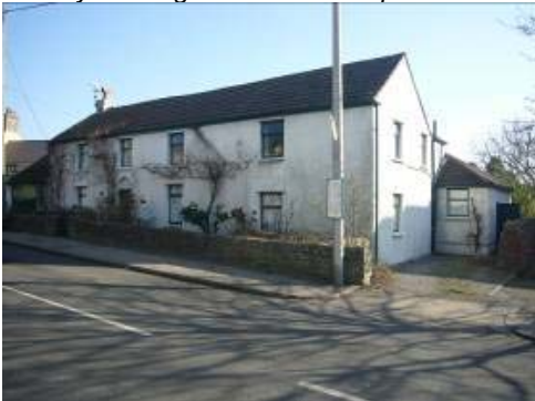
Front boundary of Upper Farm Cottages consists of a characteristic stone wall.
