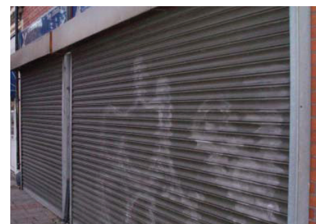
Unacceptable solid security shutters
