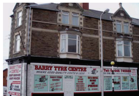
Excessive advertisements can result in a cluttered appearance.
