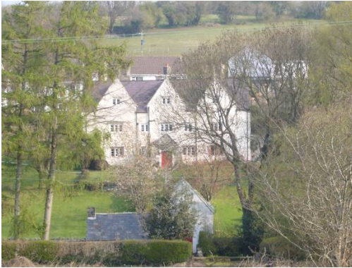
The triple gabled frontage of Great House (Grade II*).
