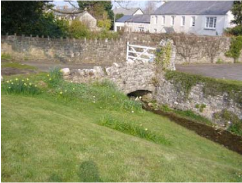
One of several stone bridges over the Nant Aberthin
