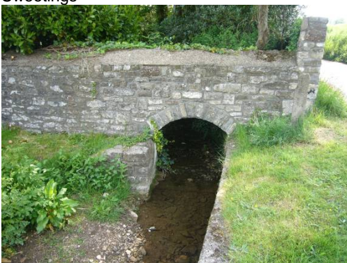
Bridge at Aberthin House
