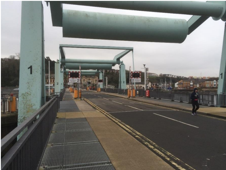
Figure 2.3: Bascule Bridges and Automatic Barriers
