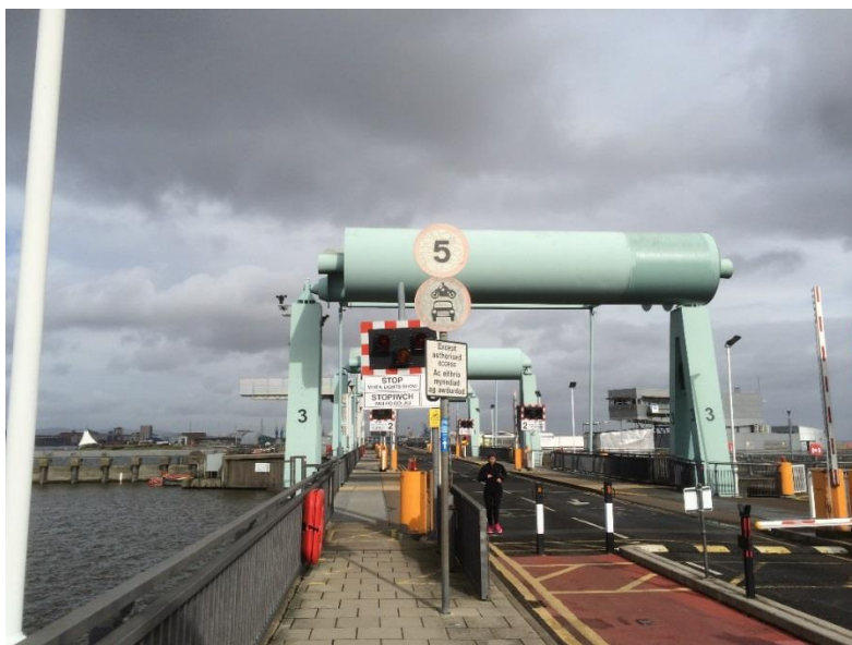
Figure 2.4: Photograph of Vehicle Access to Western End of Barrage
