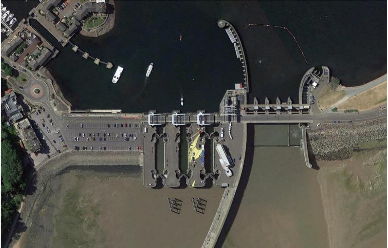
Figure 2.2: Aerial Image of Cardiff Bay Barrage Lock and Sluice Structures
