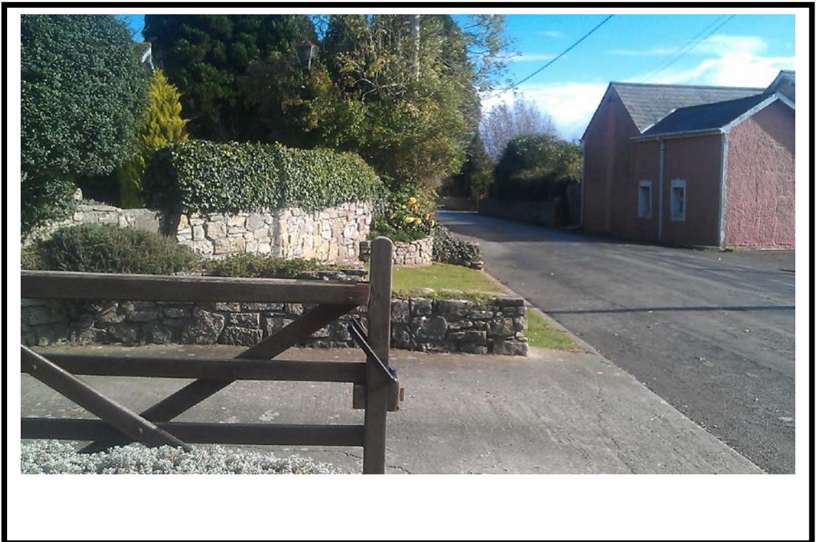
Visibility Splay in a Easterly direction along Llantwit Road from the Existing gated access / Public Right of Way with Llantwit Road located between the properties known as Wilmot and Ty Gwyn.
