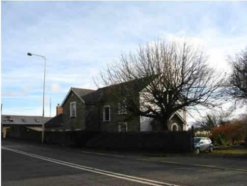
Broadway House, an unlisted but 'positive' building.
