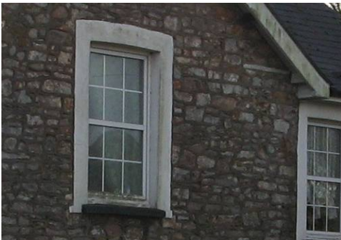
Inappropriate detailing such as the use of uPVC windows can detract from the quality of a building.
