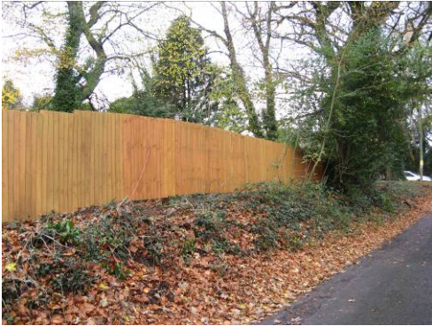
Inappropriate boundary treatments can have a negative effect on the Conservation Area.
