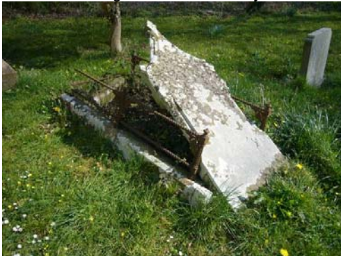
Some gravestones are in need of attention.
