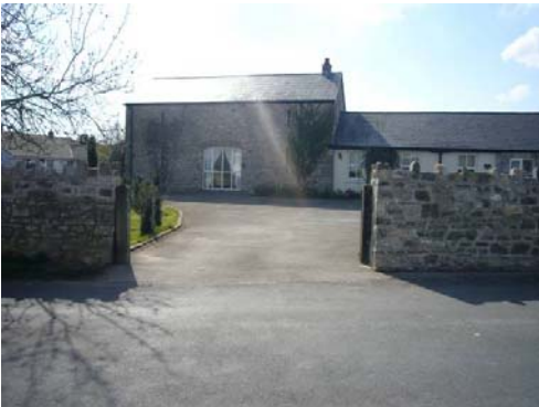
Former farm buildings, for example this granary, have been converted to residential use.
