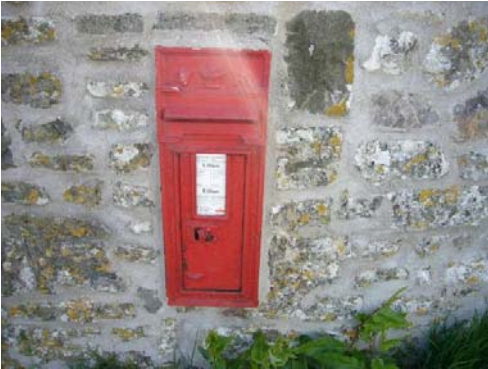
Small features such as this Victorian letter box add to local distinctiveness and should be preserved
