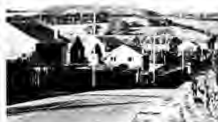
East Barry looking North to the Pencoedre Woods development area
