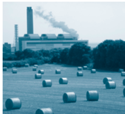
Aberthaw Power Station
