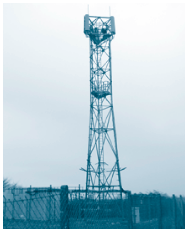
Mobile phone mast near Llandow
