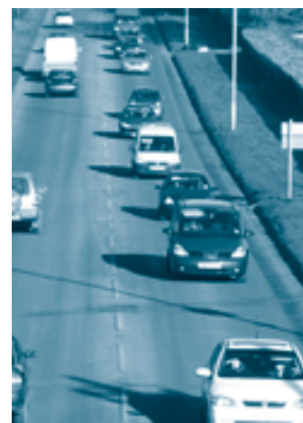
Traffic on the Barry to Culverhouse road
