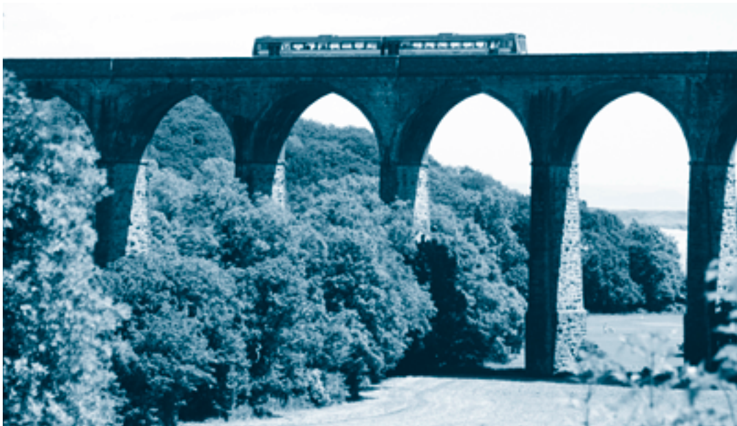
The Vale of Glamorgan Line at Porthkerry Park
