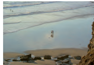
Breakwater, Barry Harbour
