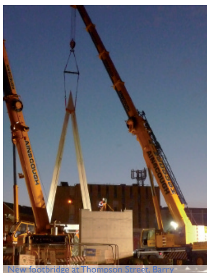
New footbridge at Thompson Street, Barry
