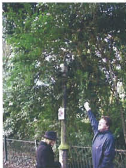
Street light (later seen illuminated) obscured by growth.
