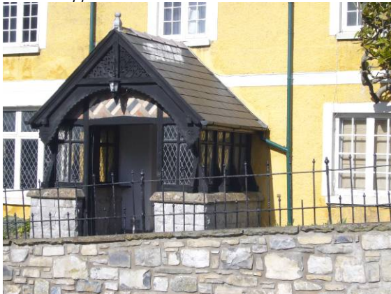
Porch and historic railings at Boverton House.
