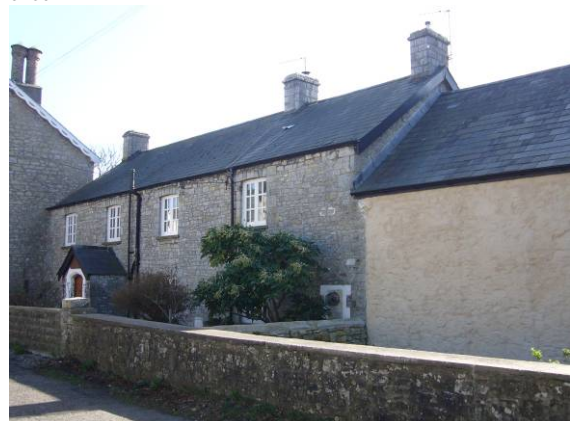
Orchard House Farm is also a 'positive building'. The attached farm buildings are now converted to residential use using appropriate materials and repair technology.
