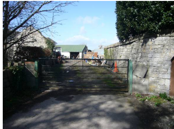
The yard near Orchard Close is not in keeping with the conservation area.
