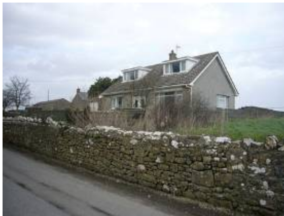
Modern infill has begun to erode the historic character of the northern group of buildings.
