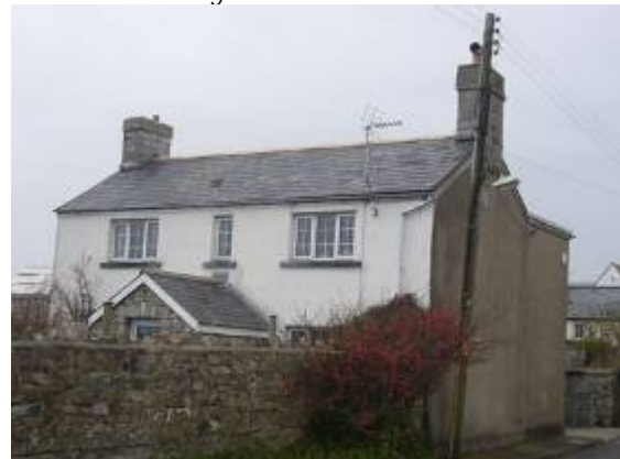
Many buildings have had their original timber windows replaced with UPVC.
