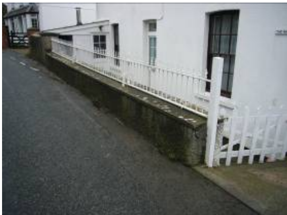
Old iron railings in front of The Manse make a positive contribution to the conservation area
