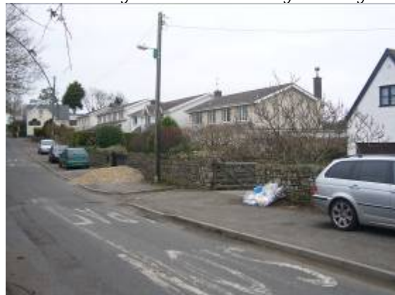
Late 20 th century linear infill is out of keeping with the historic character of the conservation area.
