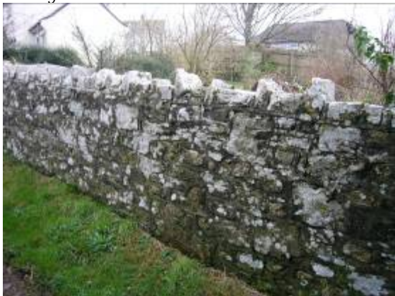
Historic roadside stone wall with a castellated coping.
