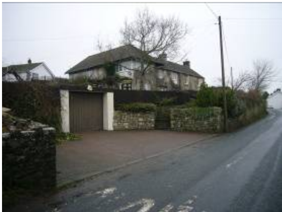
Block paving and a flat roofed garage are out of character with a historic environment.
