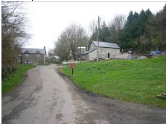
Grassed bank at the intersection of roads overlooked by Cross House.
