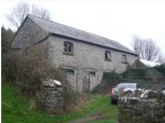
Two storey farm building.
