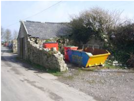
Waste and refuse might be less unsightly if concealed behind repaired stone wall.
