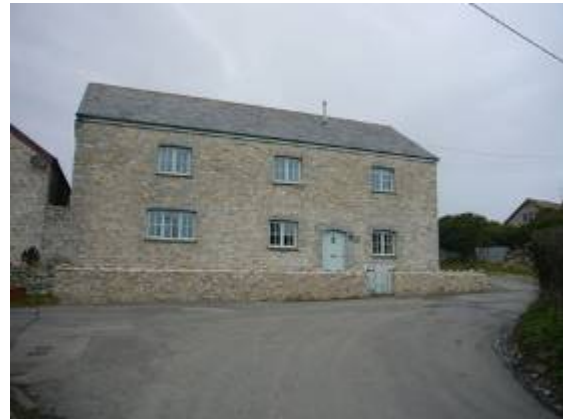
Stone building built on the site of the monastic college, Broughton
