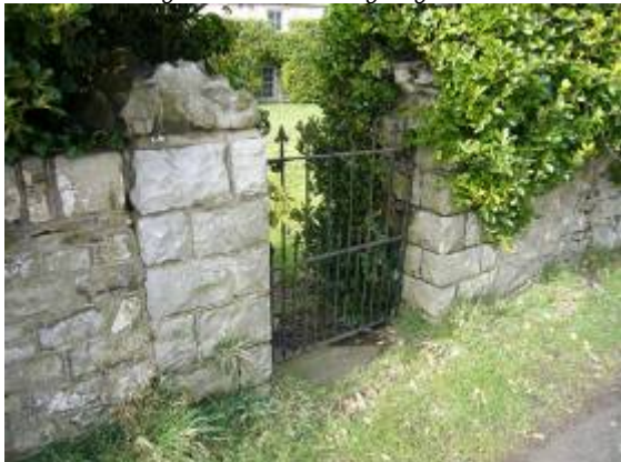
The 19 th century stone wall and gate piers of Church Farmhouse are listed grade II.
