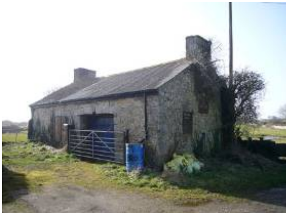
This former 19 th century forge is listed grade II.
