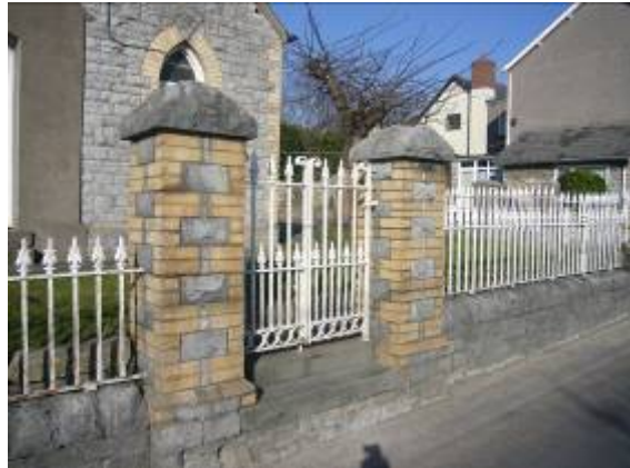
Iron railings along the front boundary of the former chapel.
