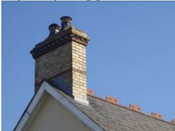
Chimney stack embellished by two tones of brick colour and ornamental courses.
