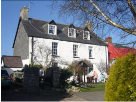
Lower Farm House is a grade II listed building dating from the mid/late 18 th century.
