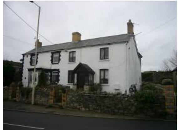
Some old buildings have lost their original timber windows.
