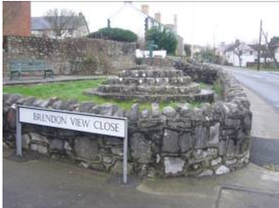
The area around the village pump would benefit from refurbishment.
