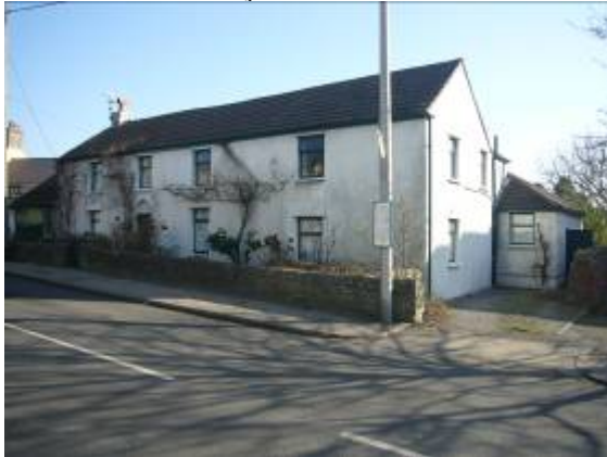
The front boundary of Upper Farm Cottages consists of a characteristic stone wall.
