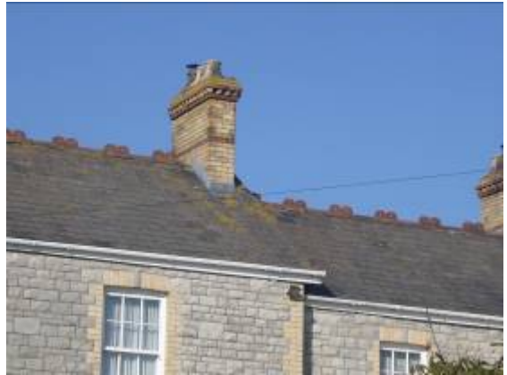
Clay ridge tiles are a feature of late 19 th century buildings
