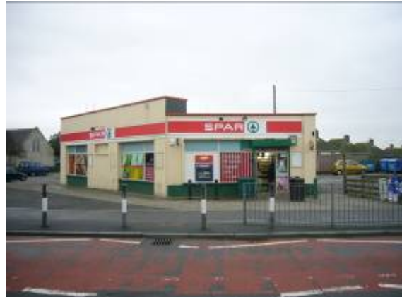
The open space in front of the supermarket is a poor area of townscape.
