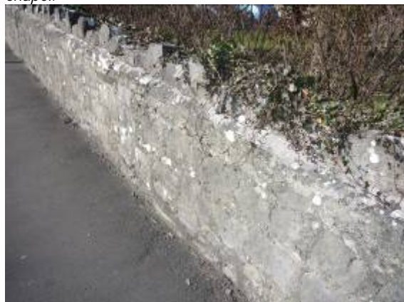
Some boundary walls along Rhoose Road have survived for over 100 years.
