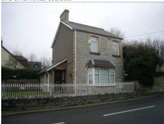
Buff brick quoins are used with the local lias building stone in this late 19 th century dwelling.
