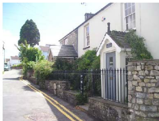
Semi private front gardens to cottages at The Limes, Cowbridge
