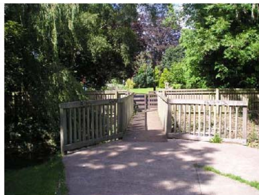
Existing footbridge over the River Thaw adjacent to The Poplars
