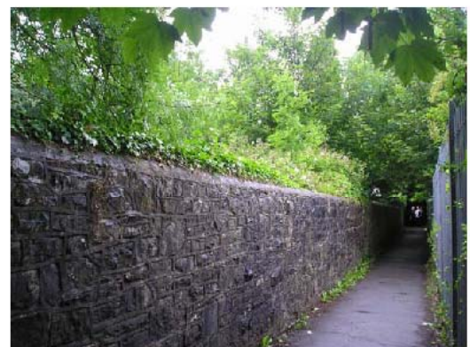
Historic stone wall along boundary of Grammar School Tennis Court
