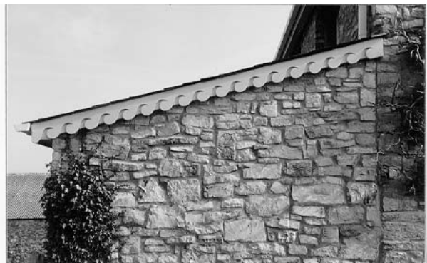
Verge detail should always be kept discreet and simple. Modern painted bargeboards do not reflect the original character of the building.
