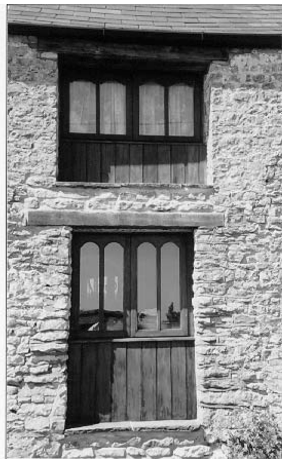
The original openings have been retained with the use of tailor-made timber window frames and panelling which blend well with the building's overall appearance.
