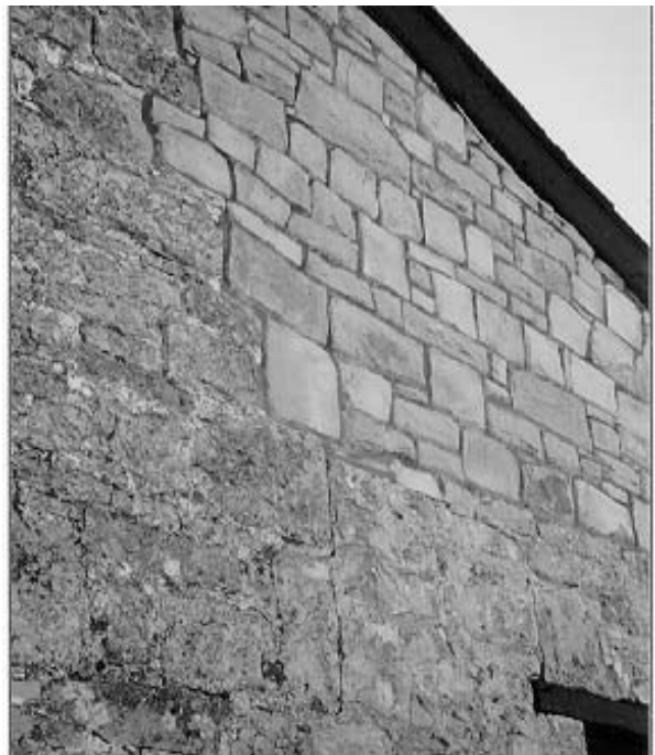
These pictures illustrate a contrast between weathered stonework with 'flush' pointing and badly restored stonework with harsh 'recessed' pointing.
