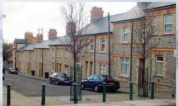
Above: External renovation of houses and environmental improvements on Harvey Street
