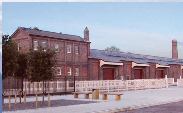
Above Right & Below: Before and after shots of the Goods Shed
