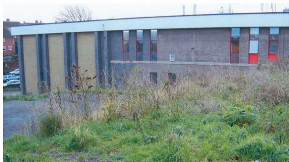
Above: Existing YMCA Building prior to commencement of works January 2005
