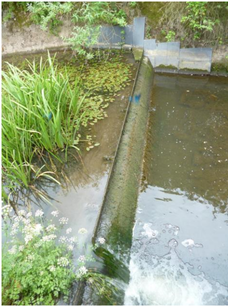
Photograph 1 - Fixed Weir Upstream
