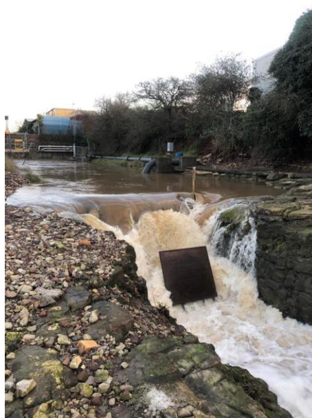
Photograph 7 – 24 th Dec View Looking Upstream Toward the Bridge
