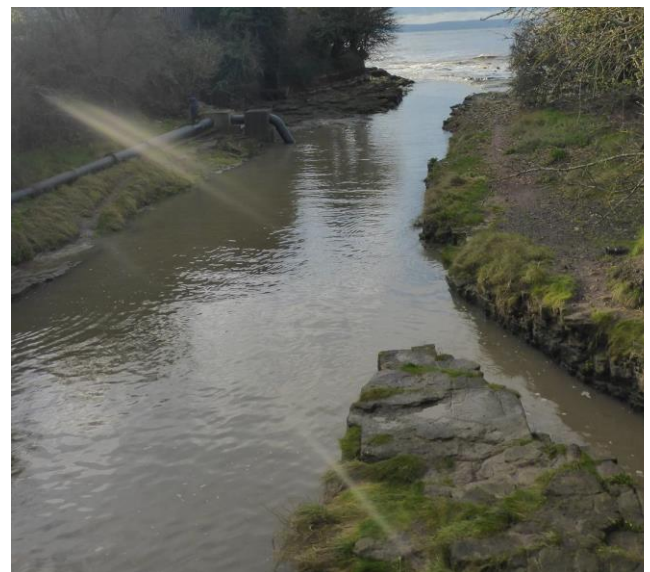
Photograph 4 - General View Looking Downstream of the Bridge
