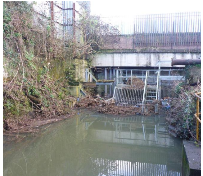
Photograph 2 - General View of the North Elevation of the Bridge
