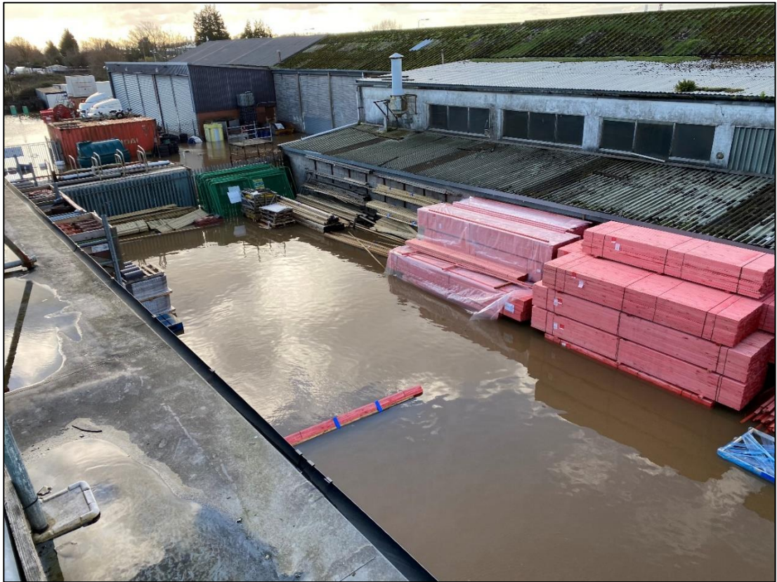
Figure 7-5: Flooding of commercial property in the north east of the area of investigation.
