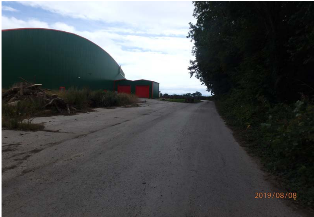
Photo 1. - proposed location of fire resistant acoustic fence along the western boundary (on outside edge / right-hand side of haul road).
