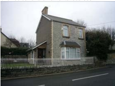
Buff brick quoins are used with the local lias building stone in this late 19th century dwelling.
