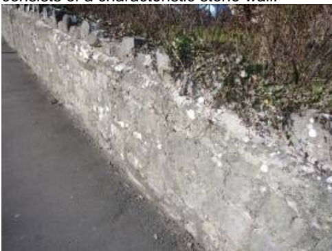
Some boundary walls along Rhose Road have survived for over 100 years.
