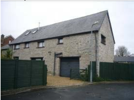
Former agricultural building at Rhose Farm now converted to residential use.
