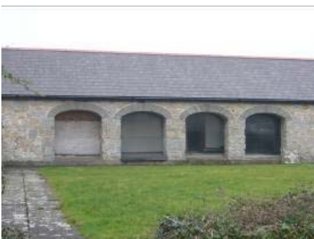
Outbuildings for agricultural equipment at Rhose Farm
