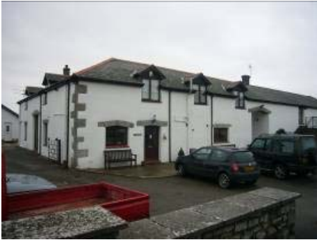
Former farm buildings at Upper Farm. Note the central carriage entrance.
