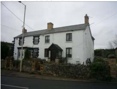
Some old buildings have lost their original timber windows.
