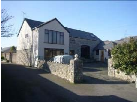
'The Granary', a converted farm building that was once part of Lower Farm.
