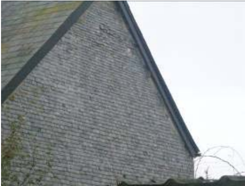
The exposed west gable of Lower House farm is given extra protection by slate hanging
