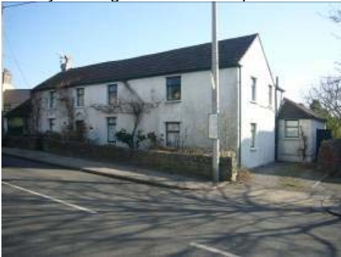
Front boundary of Upper Farm Cottages consists of a characteristic stone wall.
