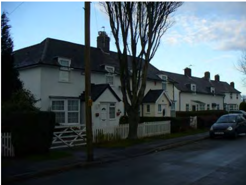
The first phase of building of the Garden Suburb on Westward Rise.
