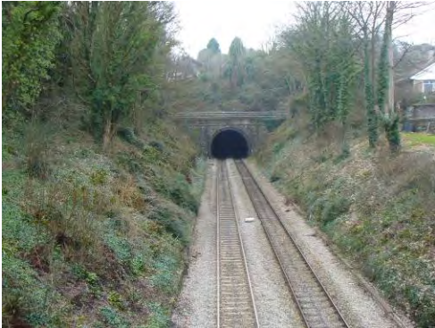
Barry Garden Suburb Railway Tunnel.
