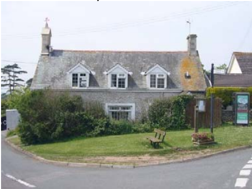
The verge of the green is being eroded by traffic.
