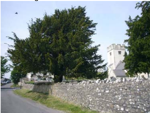
Churchyard Wall of Church of St. Michael and All Angels.
