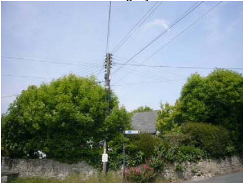
Overhead wires spoil the streetscene.
