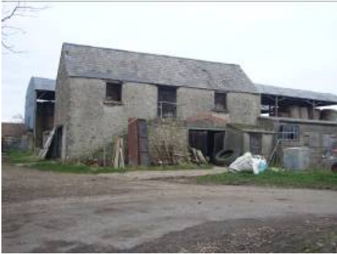
Llancadle Farm's outbuildings are built with locally quarried lias limestone.
